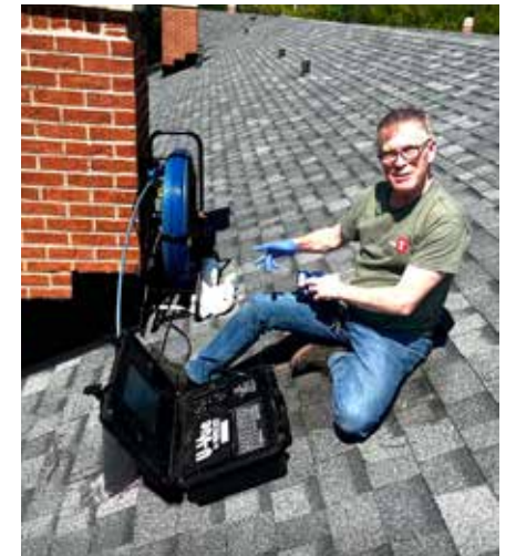
Paul LeBeau performing a rooftop sewer survey.
