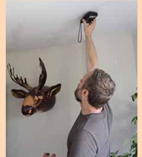
Dan Hanaway checking for moisture issues in the ceiling.
