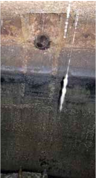
Discovered a cracked septic tank during pumping, along with a malfunctioning outlet baffle.
