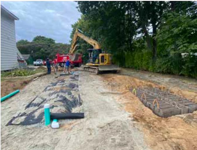
Modern leaching system installed for improved efficiency and reliability.
