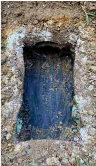
Distribution box operational but showing signs of decay.
