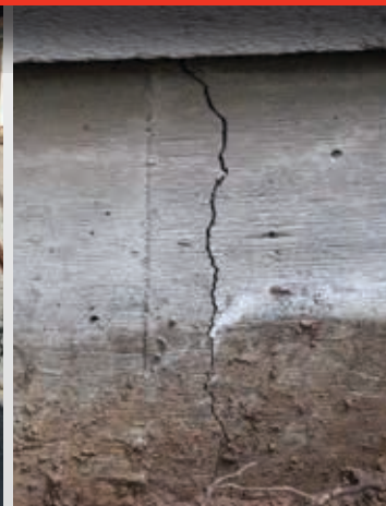
CRACKED FOUNDATION
