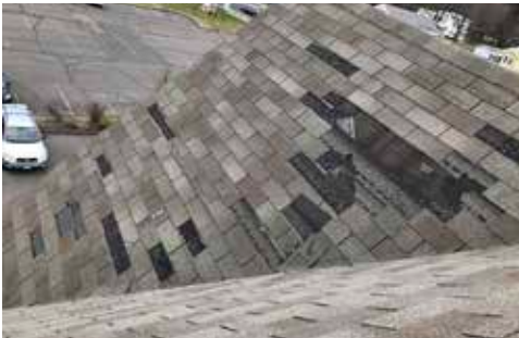
Deteriorating Shingles
