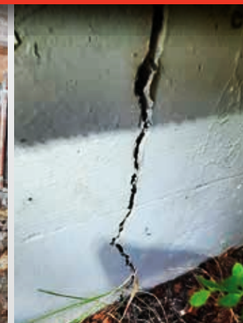
CRACKED FOUNDATION
