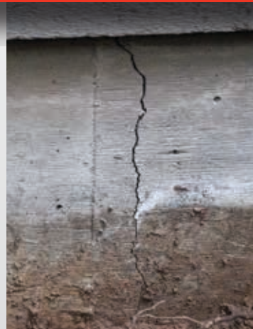
CRACKED FOUNDATION
