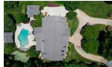
Custom Castle Roofing & Construction
