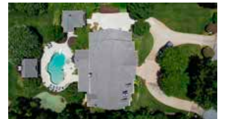
Custom Castle Roofing & Construction
