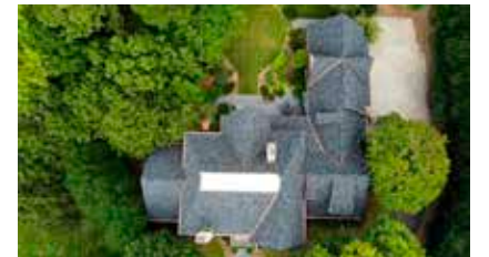
Custom Castle Roofing & Construction
