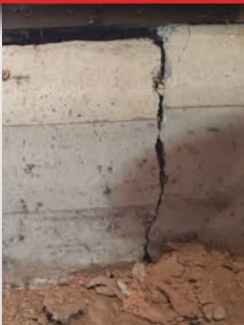
CRACKED FOUNDATION
