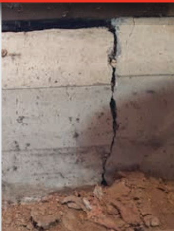
CRACKED FOUNDATION
