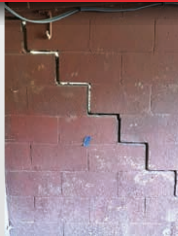
CRACKED FOUNDATION
