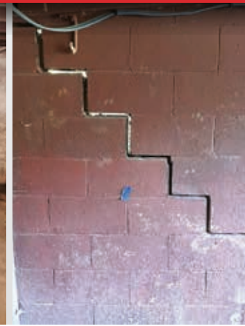
CRACKED FOUNDATION
