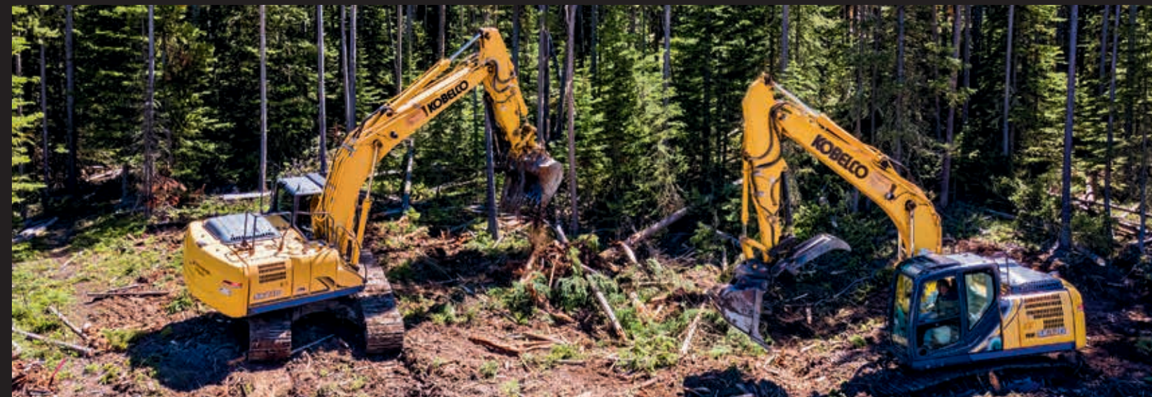
Sister company, Blaze Mountain Transport, handles all material, gravel, and ready mix concrete deliveries.
