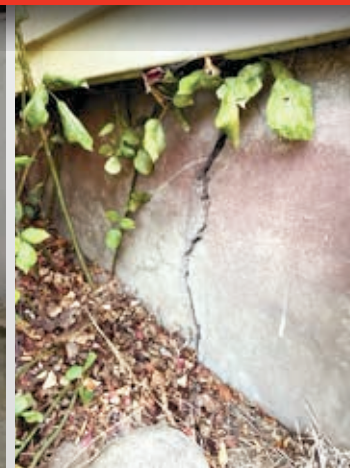
CRACKED FOUNDATION
