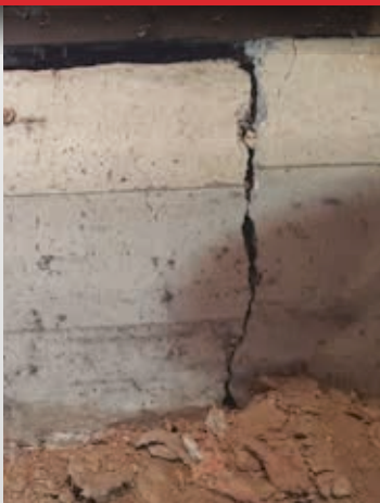
CRACKED FOUNDATION
