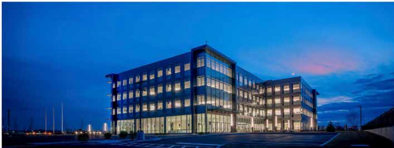
Acyo Building, Syvertsen Rigosu Architects
