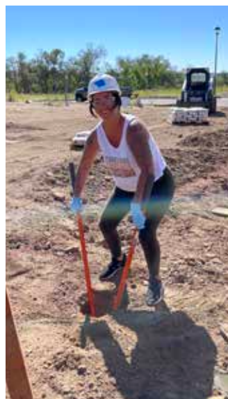
Kim Bourgois digging a post hole!
