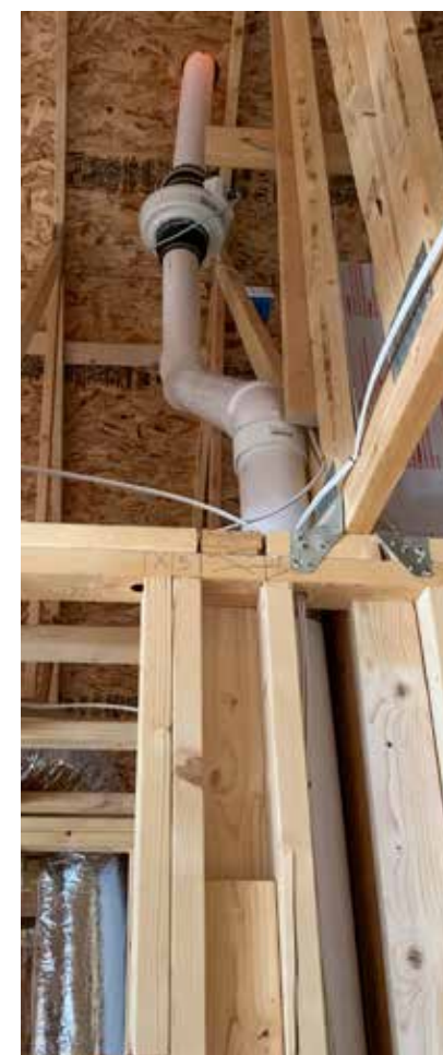
Vantage's Active Radon System
