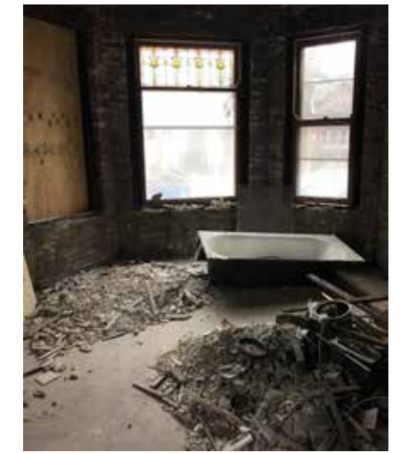
Brooke Daitchman is having her new home gutted for renovation.
