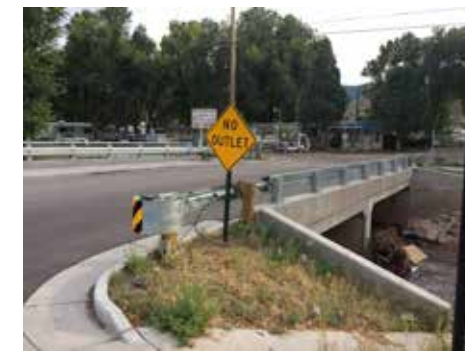
Golden Lane Bridge Replacement Over Fountain Creek
