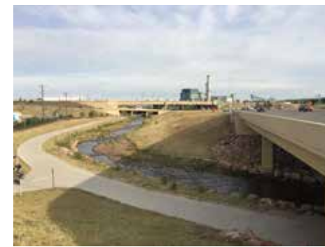
1-25 and Cimaron Interchange showing bike lane improvements
