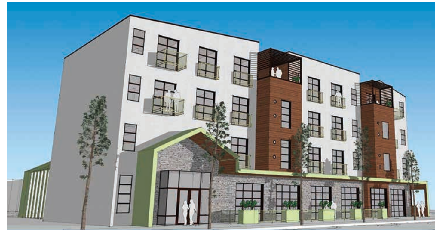
Kinship Landing, a new boutique “hostel” under construction downtown Colorado Springs. The new “cool factor” in the Springs for younger adults.
