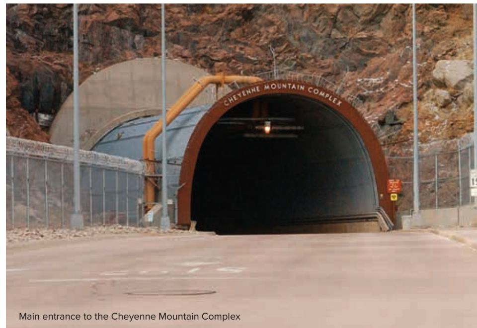
The 25-ton blast door in the Cheyenne Mountain nuclear bunker is the main entrance to another blast door (background)
