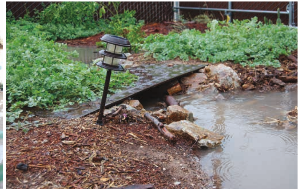
Creating passive water harvesting features, such as basins and berms, enables rain water to sink into the local water table and supports native vegetation year-round. Photo courtesy Watershed Management Group
